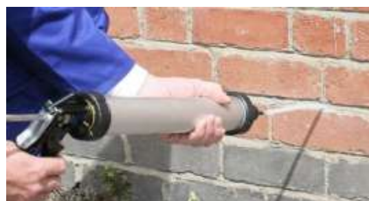
An injected DPC being applied
