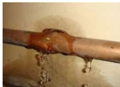
A common cause of mould growth
