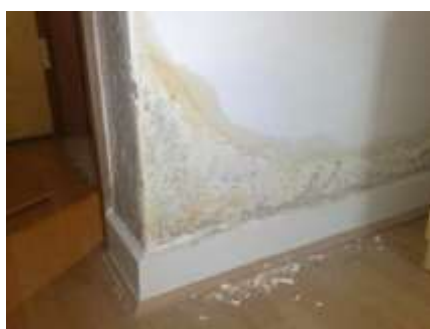
Rising damp due to failing DPC
