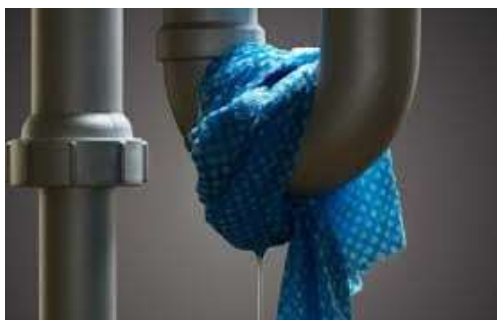
Leaking pipes a common source of moisture
